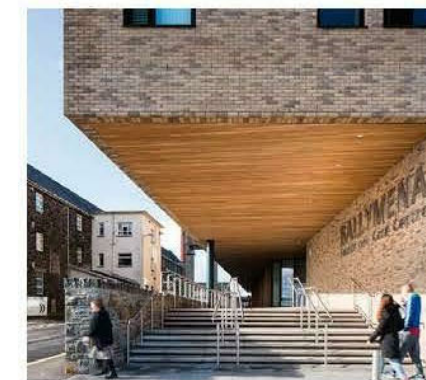
TIMBER SOFFIT TO TERRACES + PODIUM
